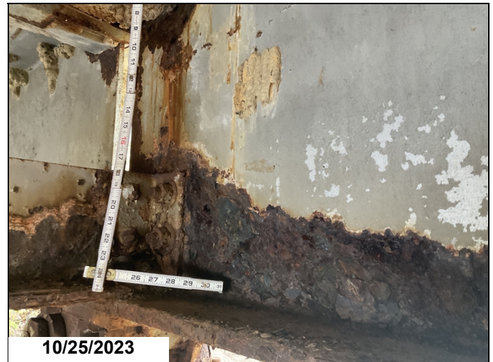
Bent 2 span 1 beam 4 at bearing area has moderate pitting to web and lower flange. Upper web at haunch area has 5/16" pitting in the upper web. Lower web above bearing has a 1/4" pitting. Lower flange has 1/16" pitting.
