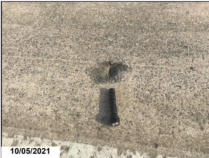
Span 2 spall
