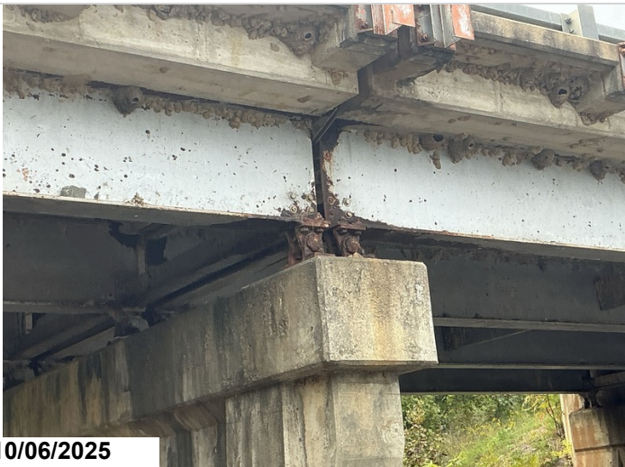
Bent 2 span 2 beam 1 has moderate pitting to the lower web and flange above bearing.
