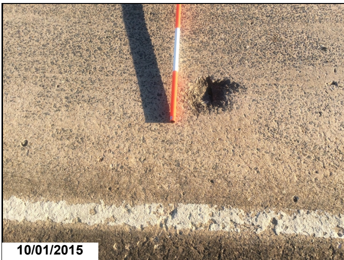
Span 2 spall in the deck.
