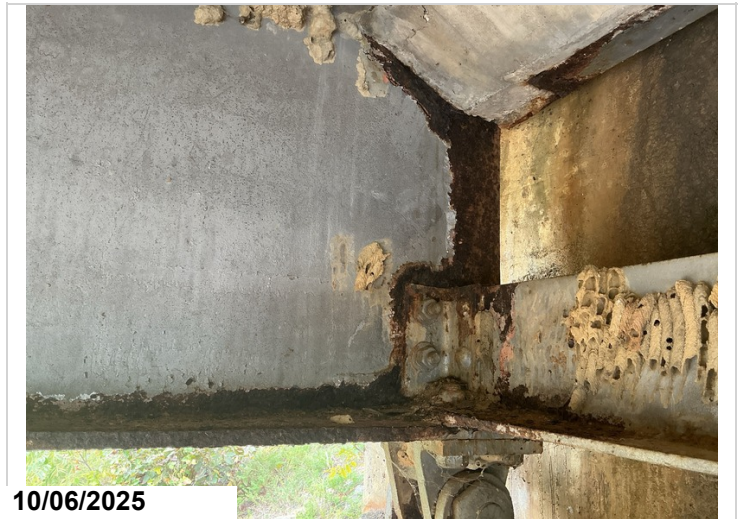
Bent 1, girder 4: section loss to the the beam end near the haunch and the lower flange. CS3-2'
