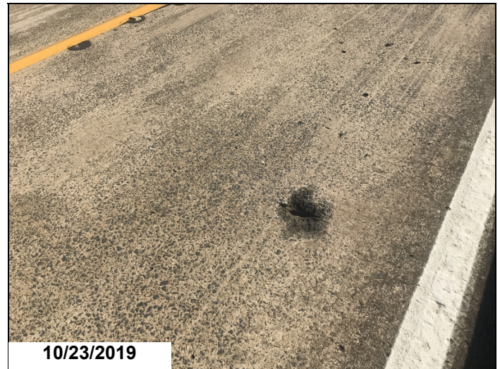
Span 2 spall
